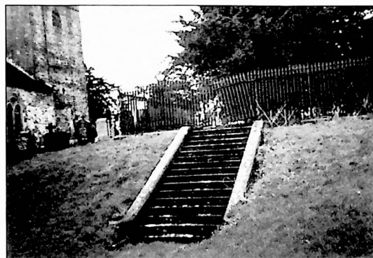
Fig. 5. View of the Adams family vault at St. David's Church, Llanarthne. A number of the steps slide outwards allowing access to the vault.
